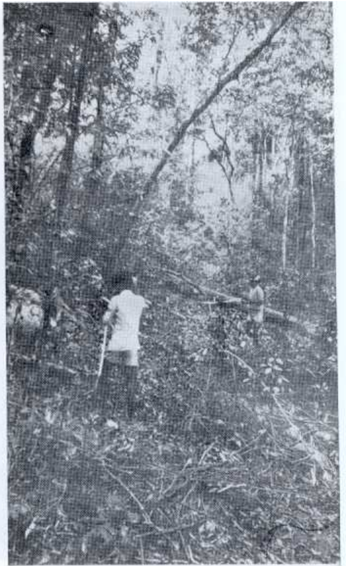
Pl. XXIX. Road laying process
