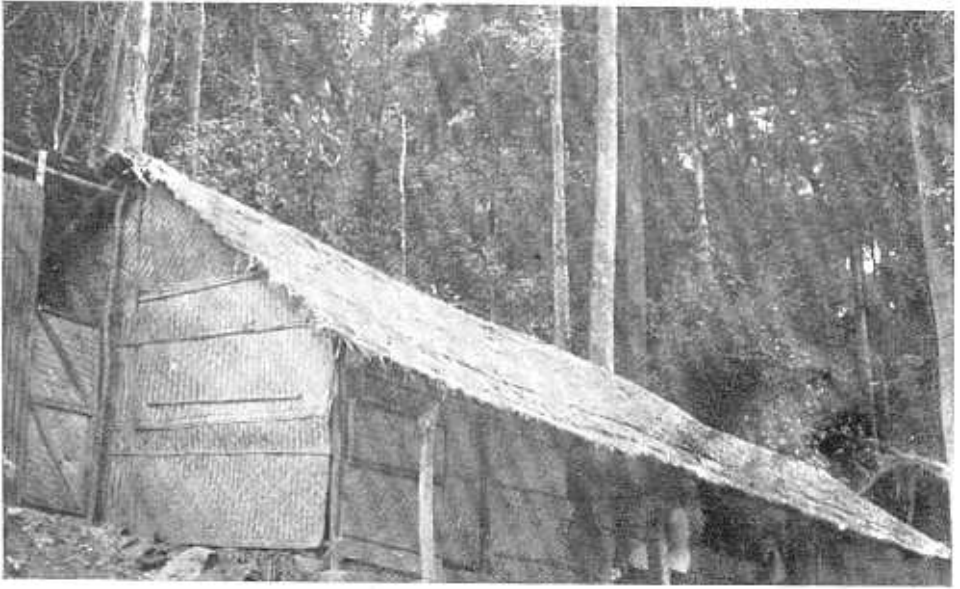
Fig. 21 Worker's Camp Shed in Silent Valley
