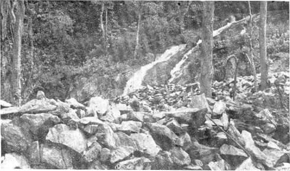
Fig. 19 Road construction in progress - A troop of Liontailed macaque was seen here
