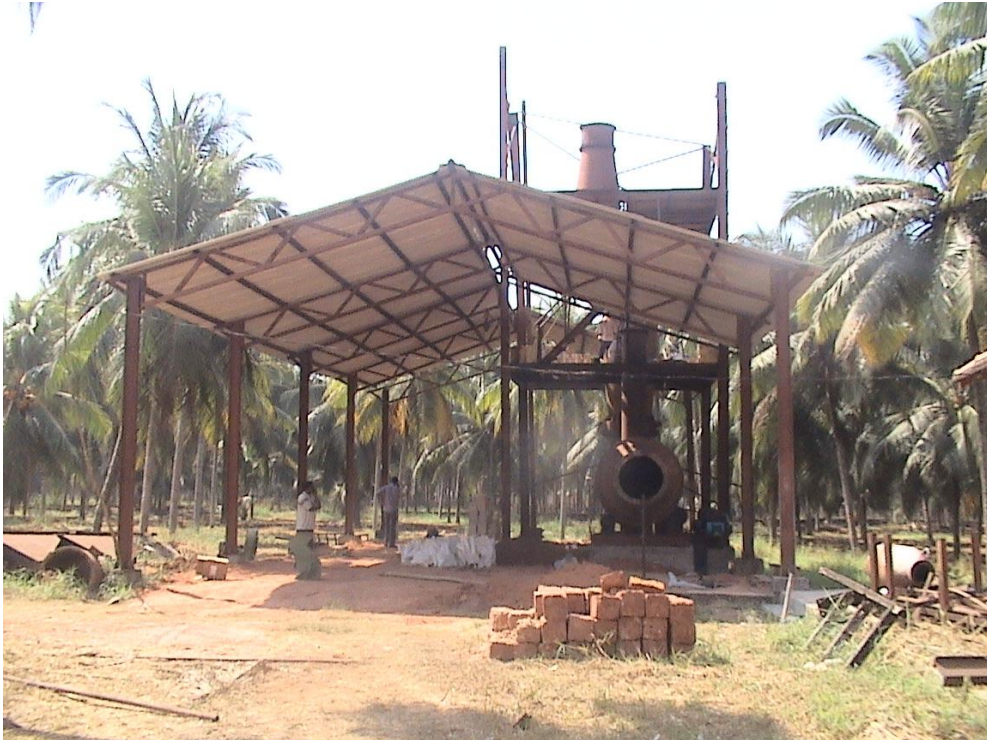
Front view of the constructing plant
