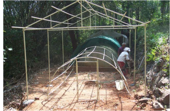
Views of Poly tunnel construction
