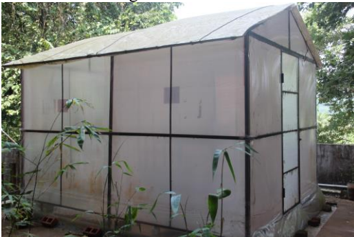
Figure 9. : Outdoor culture room made of polycarbonate.
