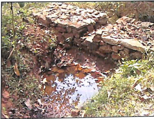
Plate 15. Water stored at check dam
