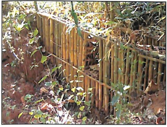
Plate 4. Bamboo check dam
