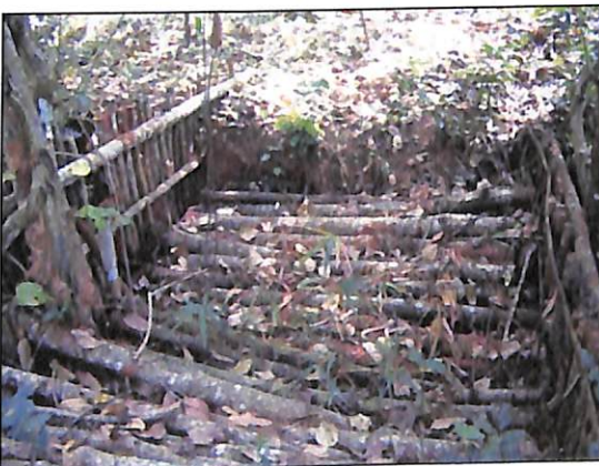
Plate 5. Dry log check dam
