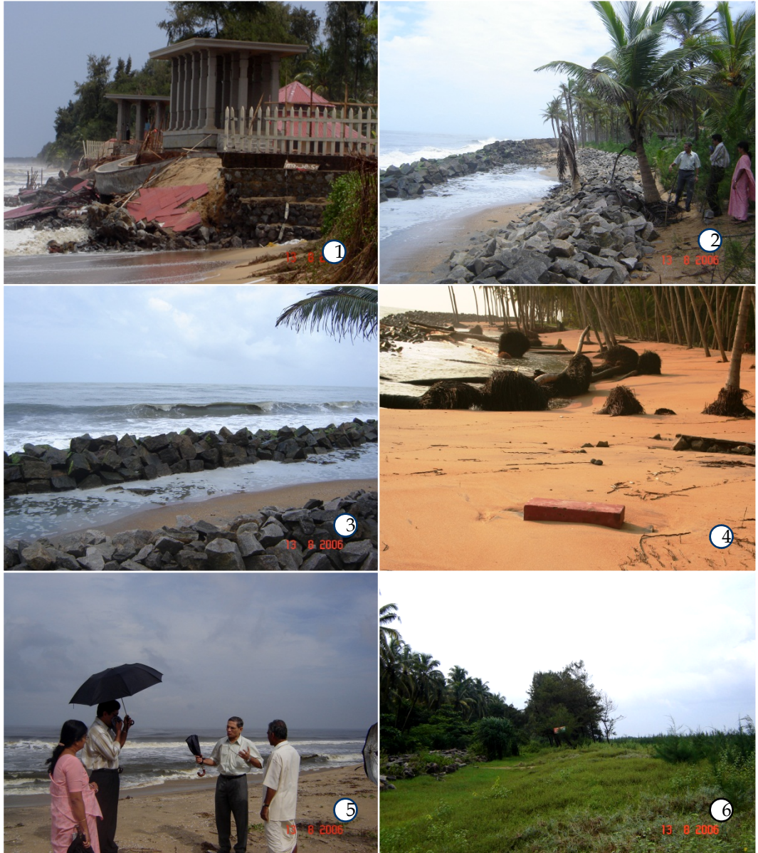
Fig 18. Damages due to waves 1. Buildings, 2 & 3 Sea walls, 4. Coconut Plantation. 5. Visit of Experts to the affected areas 6. Selected area for experimental planting of bamboo at Munackal, Eriyad Panchayath
