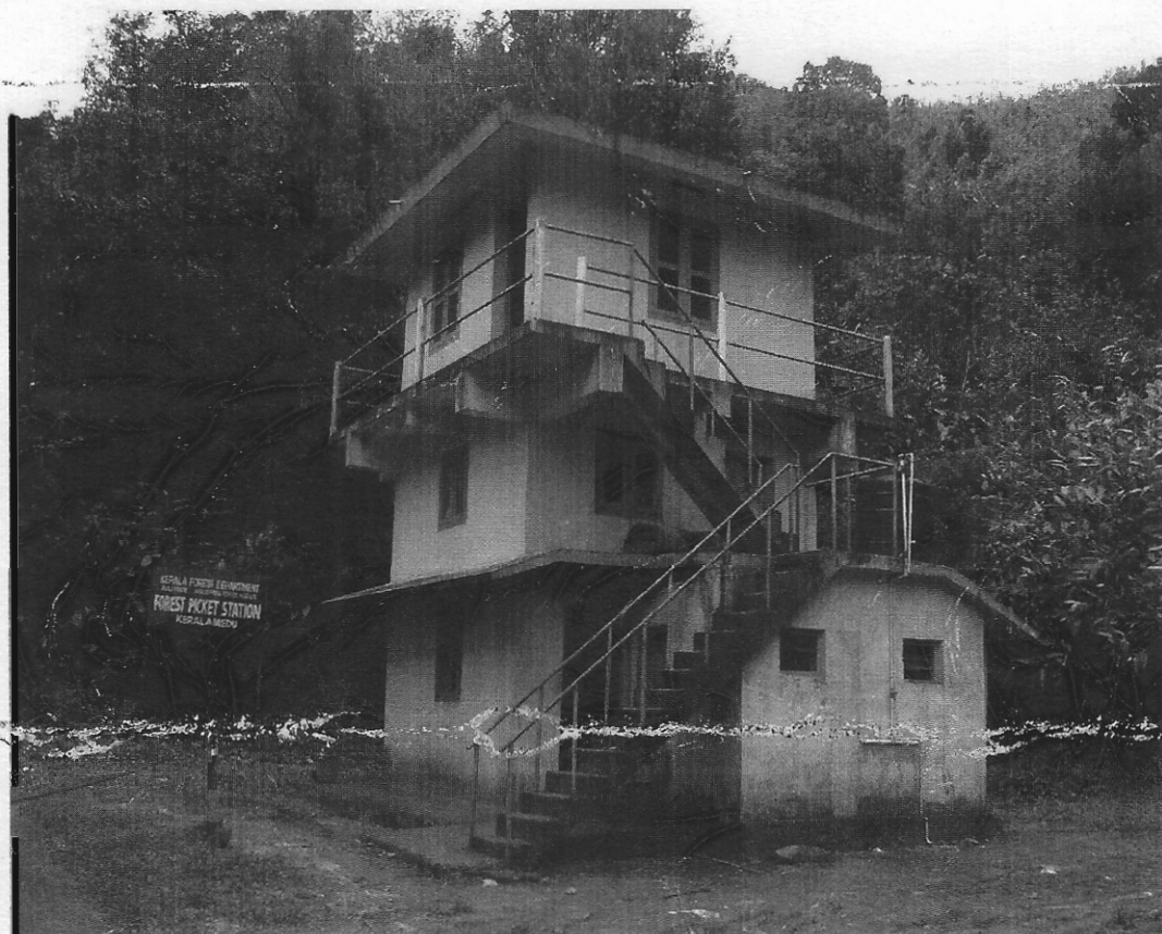
Plate 9. Singappara Forest Station (above); Keralamedu Forest Picket Station (below)
