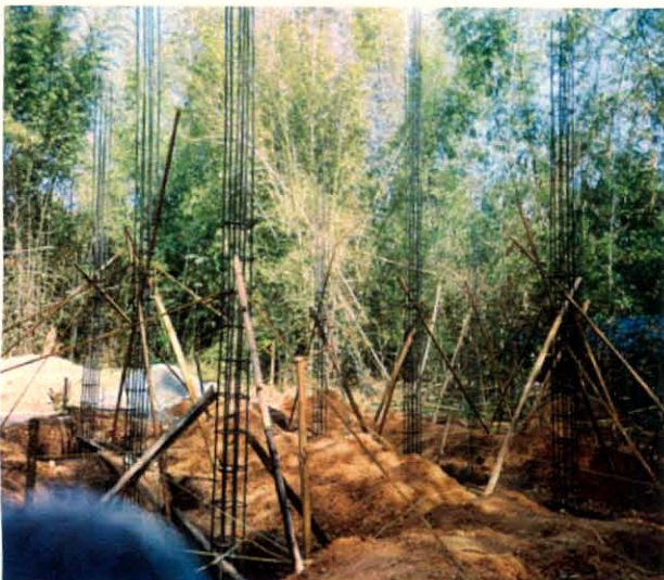
Fig. 15. Construction stages – Initial activities: Site preparation, bamboo collection, earth work, construction of columns, etc
