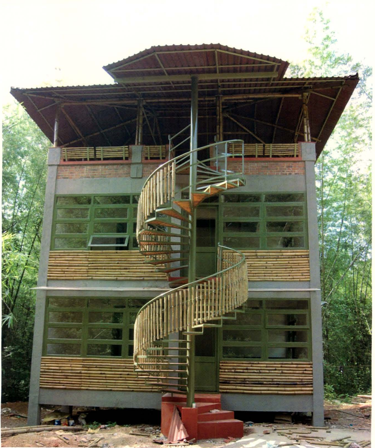
Fig. 20a. Front view of the completed bamboo house
