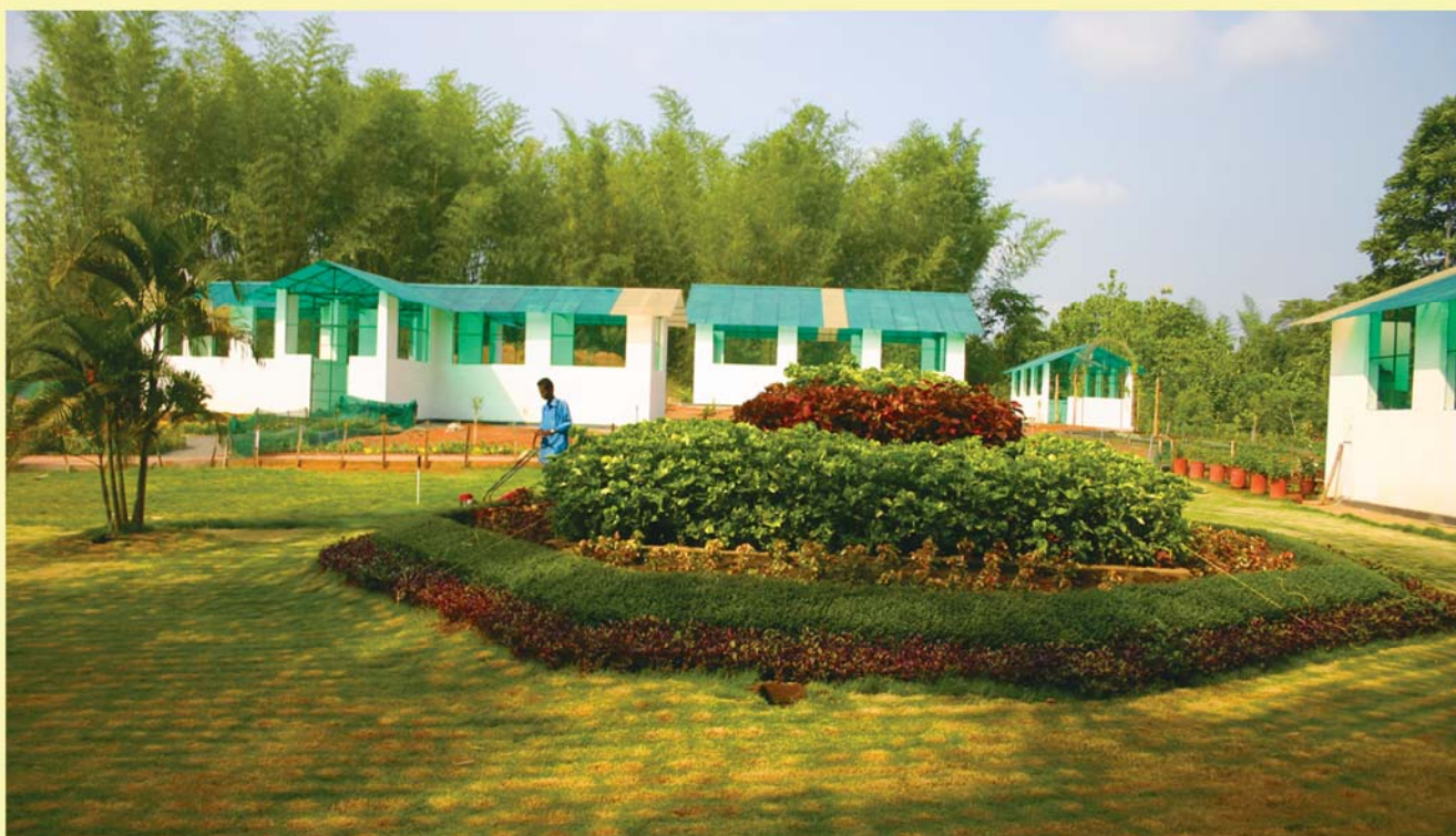
Figure 3. Thematic Houses before renovation
