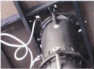
Fig 34. Air supply arrangements (air rings)
