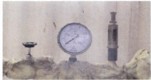
Fig. 43. Steam pressure gauge
