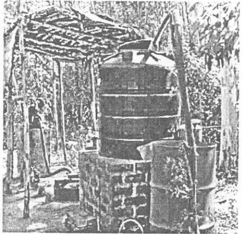
Fig. 11. Water tanks and pump - part of misting system
