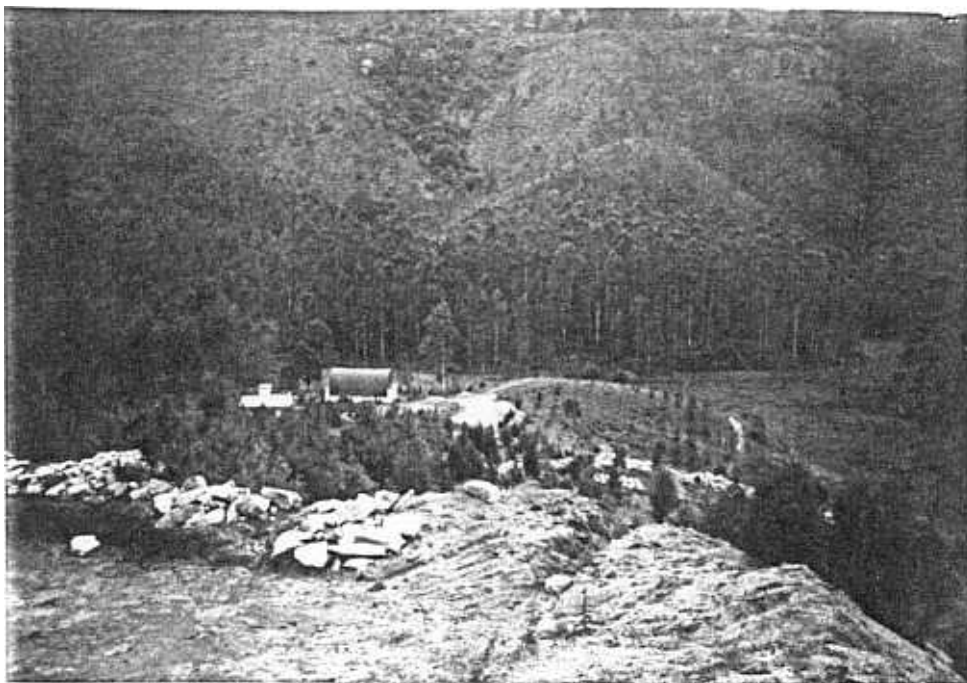
View of the sanctuary from Northern side during the zig-zag construction of the road
