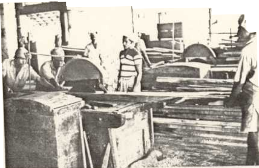
Fig 10 Circular resaw
