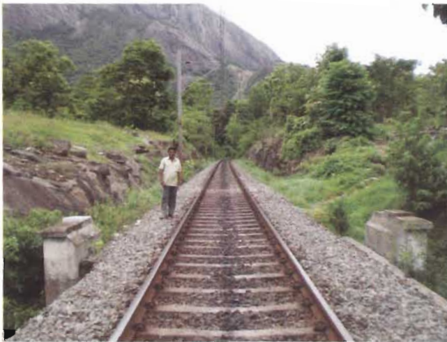
Figure 1. Railway track with narrow sideways
