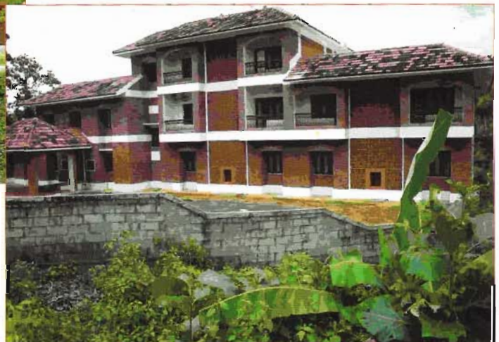
The Trainees Hostel – Provides modern boarding and lodging facilities to trainees and guests. Has 12 a/c double rooms, 4 non a/c rooms, two dormitories each with 25 a/c cubicles.
