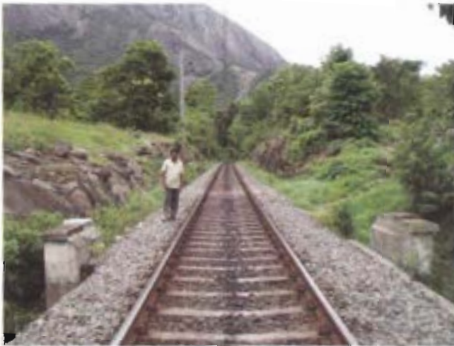
Figure 1. Railway track with narrow sideways
