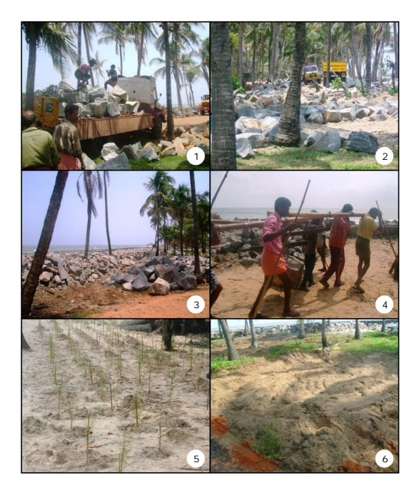
**Plate 8**. 1-4. Different stages of sea wall construction. 5 & 6 The planted area before and after sea wall construction.
