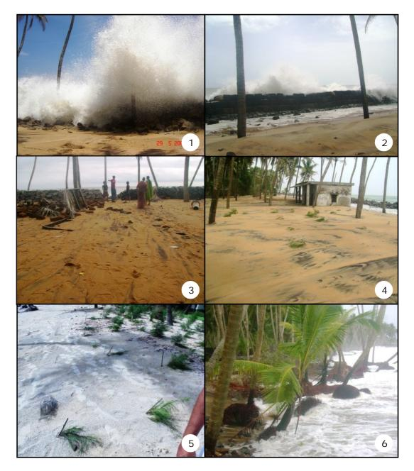
**Plate 9**. A view of the raising waves during high tides 2. Waves thrashing above the sea wall and flowing water behind the wall resulting in sand erosion 3. Sea water flows through the damaged area of sea wall. 4 & 5. Sand deposited on the shore above *Casuarina* seedlings. 6. A view of the damage to coconut trees due to high tides.
