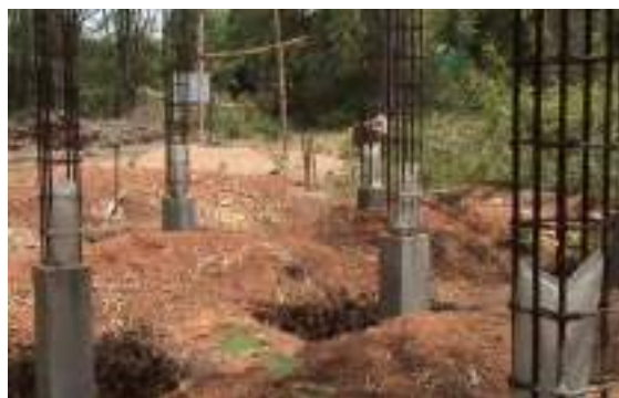
Construction of bamboo house
